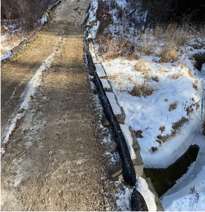
Fig 1: Temporary mat bridge over stream DS46 between Strs. 51 & 52. Viewing northeast. (12-26-19).
