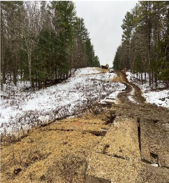
Fig 7: Foundation can set in place for Str. 53. Viewing southwest. (12-27-19).
