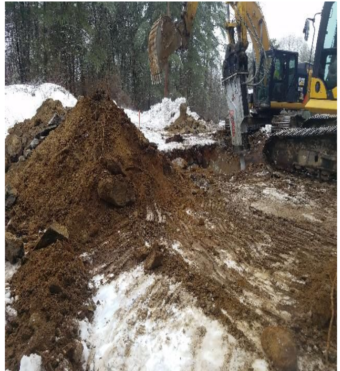
Fig 12: Crew hammering ledge for foundations at Str. 55. Viewing southwest (12-31-19).
