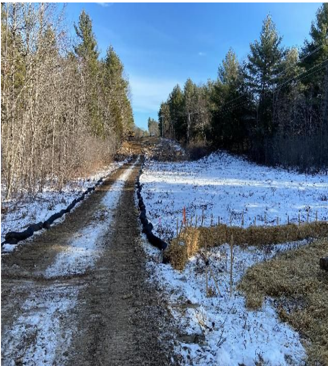
Fig 3: Installed siltation controls at wetland DW33 crossing. Viewing east. (12-26-19).
