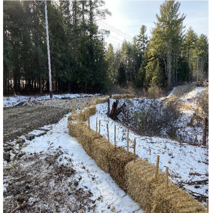
Fig 2: Straw bales installed upslope of stream DS46. Viewing southwest. (12-26-19).
