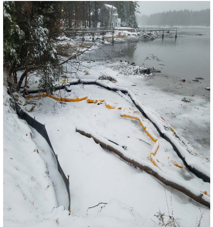
Fig 8: Turbidity barrier installed in intertidal zone at Gundalow landing/ east side of the Bay. Viewing south. (12-30-19).
