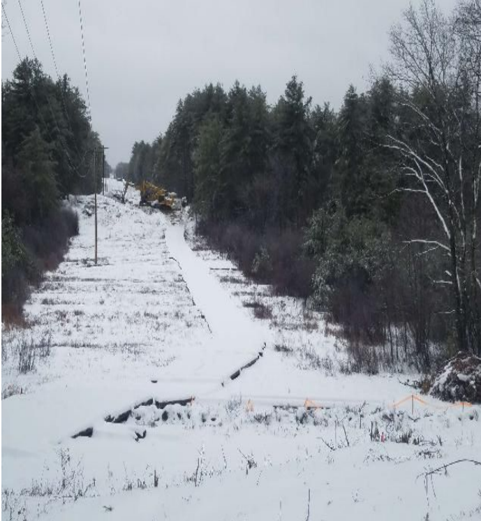
Fig 13: Temporary matted access road through wetland DW31 between Strs. 55 & 56. Viewing southwest. (12-31-19).
