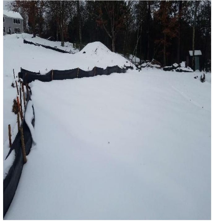
Fig 10: BMPs installed on slope at Getchell property/west side of the Bay. Viewing north. (12-31-19).
